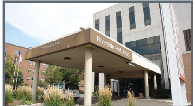
RIVERSIDE MEDICAL BUILDING Minneapolis, MN
