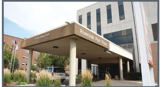
RIVERSIDE MEDICAL BUILDING Minneapolis, MN
