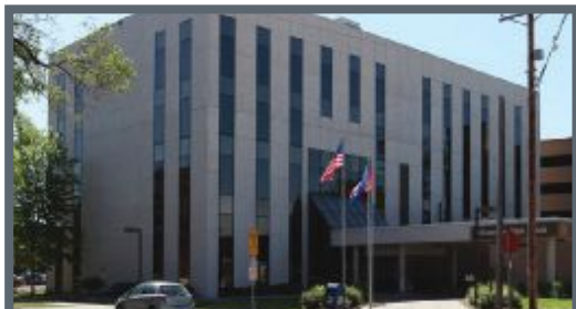
RIVERSIDE MEDICAL BUILDING Minneapolis, MN
