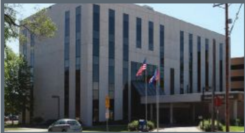
RIVERSIDE MEDICAL BUILDING Minneapolis, MN
