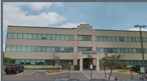
RIDGEVIEW MEDICAL BUILDINGS Burnsville, MN
