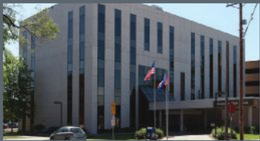
RIVERSIDE MEDICAL BUILDING Minneapolis, MN
