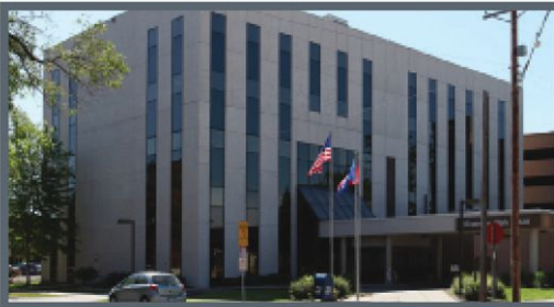
RIVERSIDE MEDICAL BUILDING Minneapolis, MN
